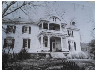
Recent photo – Eastern View on Clark's Mountain Road, built in 1839, has had major renovations recently and over its long history. It was Ogden Halsey's home. He was a descendant of Benjamin Walker (See next page) as were we and thus Ogden was our cousin.
